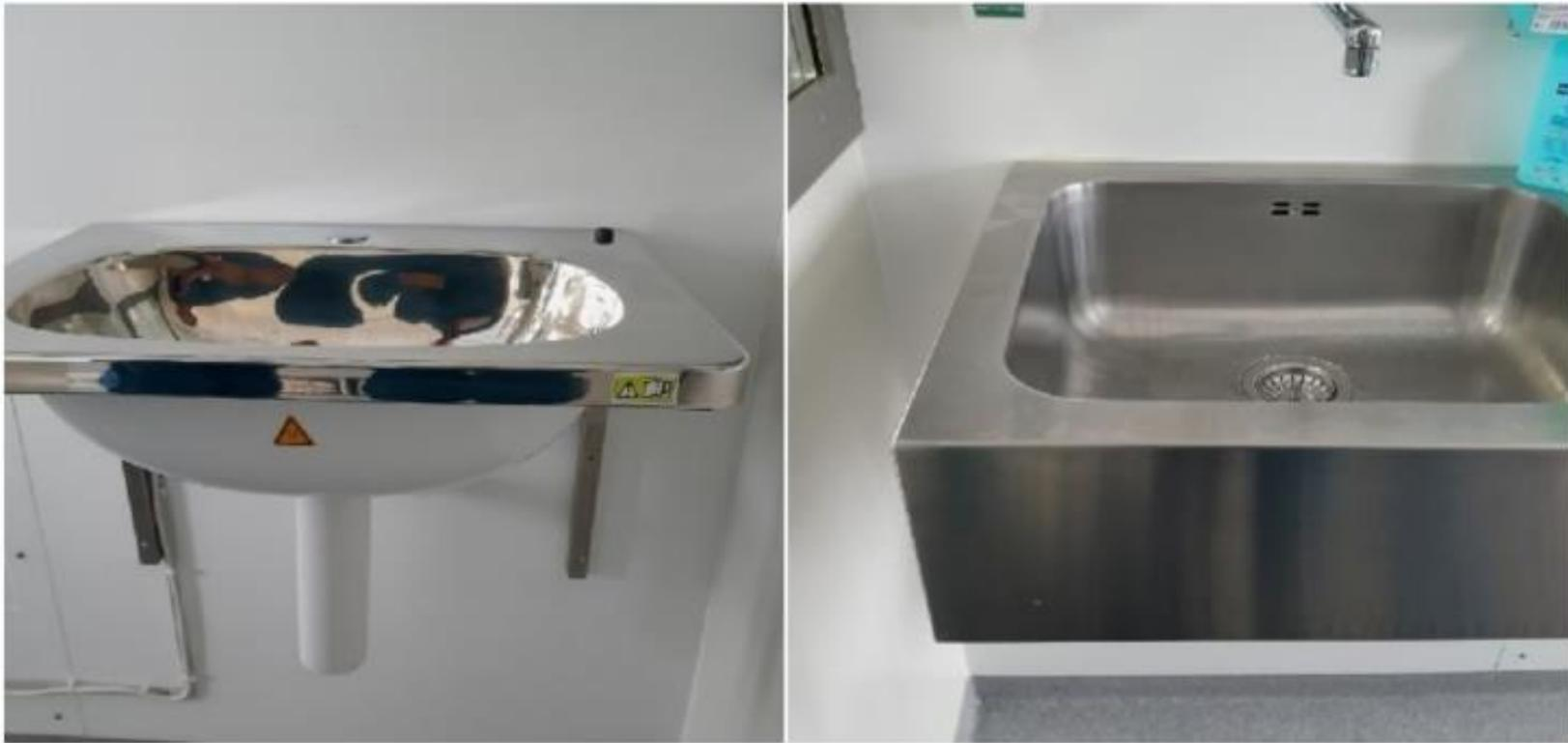
**Figure 1.** The self-disinfecting sink installed in room 1 is shown to the left, whereas the regular sink used in all of the other rooms in the Burn Centre is shown to the right.
