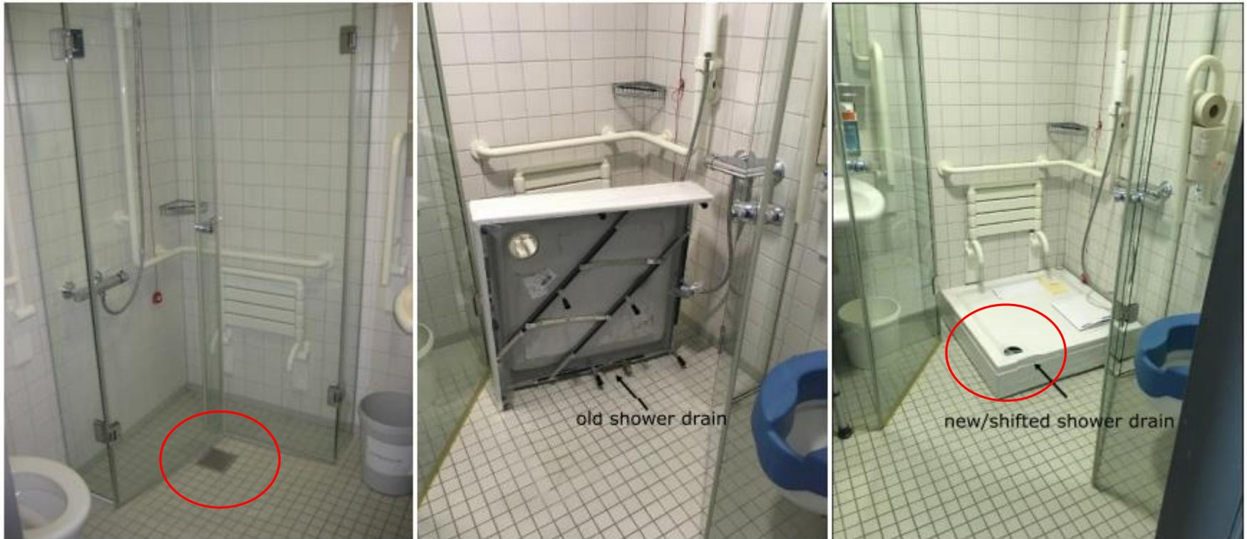
**FIG 6** Removable and autoclavable shower insert to prevent direct contact with wastewater. Following unsuccessful eradication and new detections, removable shower tubs were installed to avoid backsplash by shifting the shower drain away from the water jet from shower heads.
